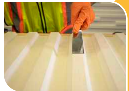
Screeding caulk with putty knife on smooth rib
