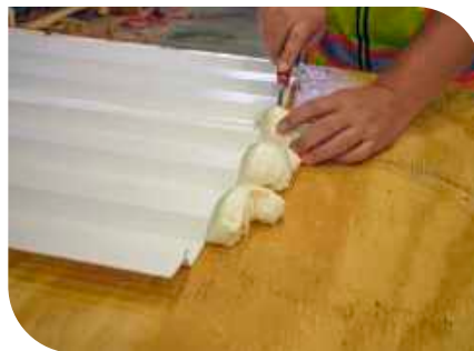
2. Allow the foam to ooze out and harden
