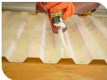
Sealing formliner with caulk at seam
