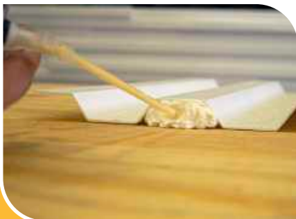
1. Apply spray foam in gap
